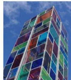
GLZ-2: BLUE LAMINATED GLASS, SAFLEX & VANCEVA COLORS PVB INTERLAYERS
